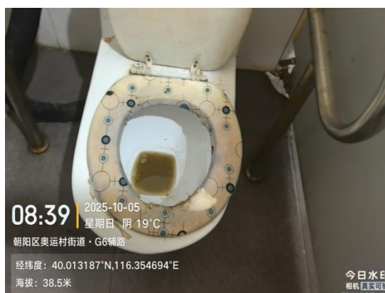
清河收费站(洗手池破损)T08:40
